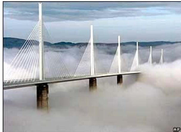
Cable-stayed bridge over the River Tarn.
