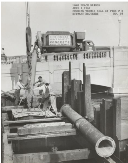
Workers pouring tremie seal at Pier # 2, 1954
