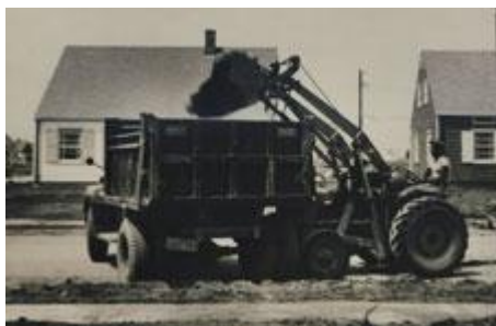
Loader emptying dirt into a dump truck, c.1948
