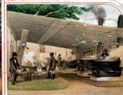
COOKING DEPARTMENT, S.W. COR. WASHINGTON AVE. & SWANSON ST.
