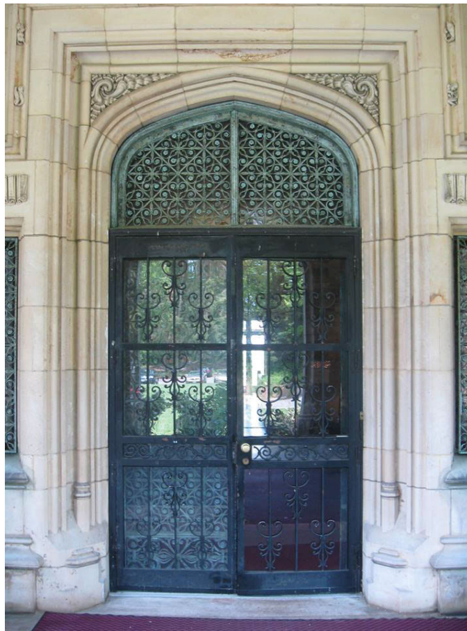
Inisfada, front door-closeup, May 2013
