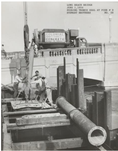
Workers pouring tremie seal at Pier # 2, 1954
